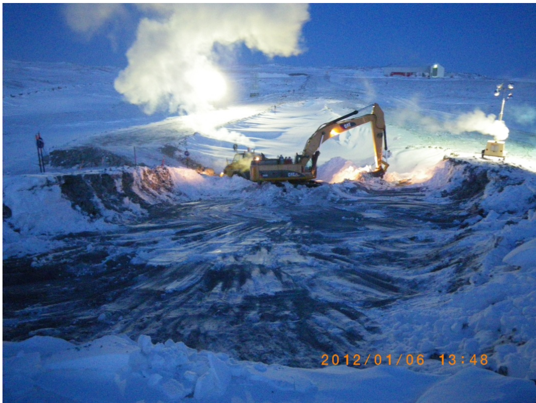
Photo 1: Removal of snow from the North Dam over the keytrench. Looking east from the west side of the North Dam keytrench.
